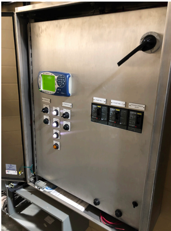
The MultiSmart® iPSMs provide Suffolk County a sophisticated technology that can collect data and alarm control system alerts from their stations, and prioritize issues that truly require a technician call-out.
