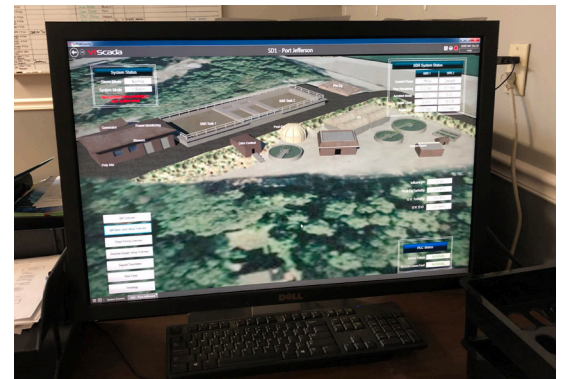
Suffolk County DPW implemented the next generation of Xylem's Flygt Outpost SCADA system to more proactively manage their sewer system and better manage their inventory.
