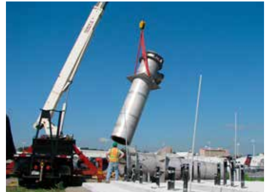
Installation of Flygt submersible pumps at LaGuardia airport.
